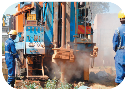
The borehole being drilled
